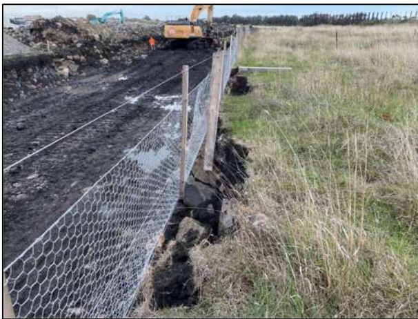
Plate 41. Erosion of offset site adjoining construction area (Ecology and Heritage Partners Pty Ltd 31/05/2023).
