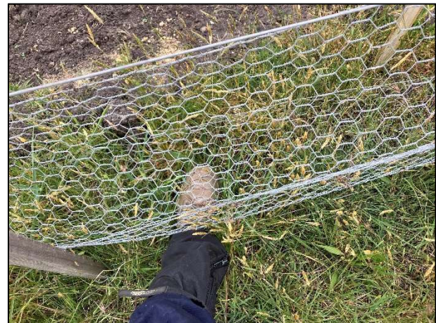
Plate 32. Gap underneath eastern fence rabbit proofing (Ecology and Heritage Partners Pty Ltd 01/11/2023).
