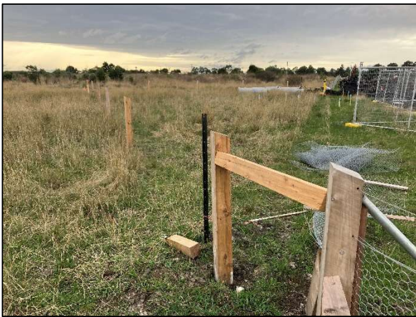
Plate 29. South-eastern fence being corrected to intended alignment (Ecology and heritage Partners 31/05/2023).
