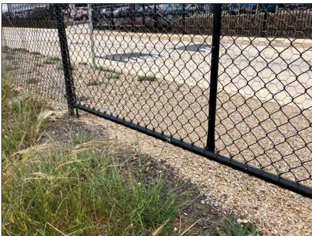
Plate 37. Rabbit proofing on bottom of reinstated gate (Ecology and Heritage Partners Pty Ltd 02/11/2023).
