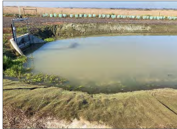
Photograph E2 – Drainage line and retarding wall immediately adjacent to the south and south-east border of the study area.
