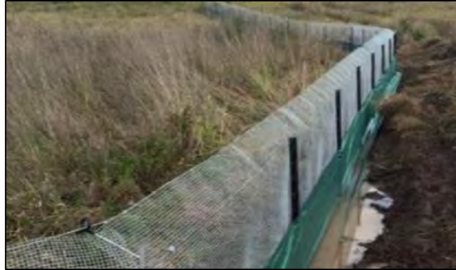
Plate 8. Example of suitable frog exclusion fencing (fence posts must be on the outside and not within the Offset Area)
