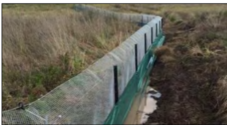
Plate 8. Example of suitable frog exclusion fencing (fence posts must be on the outside and not within the Offset Area)
