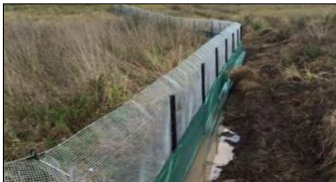
Plate 3. Example of suitable frog exclusion fencing (fence posts must be on the outside and not within the Offset Area)
